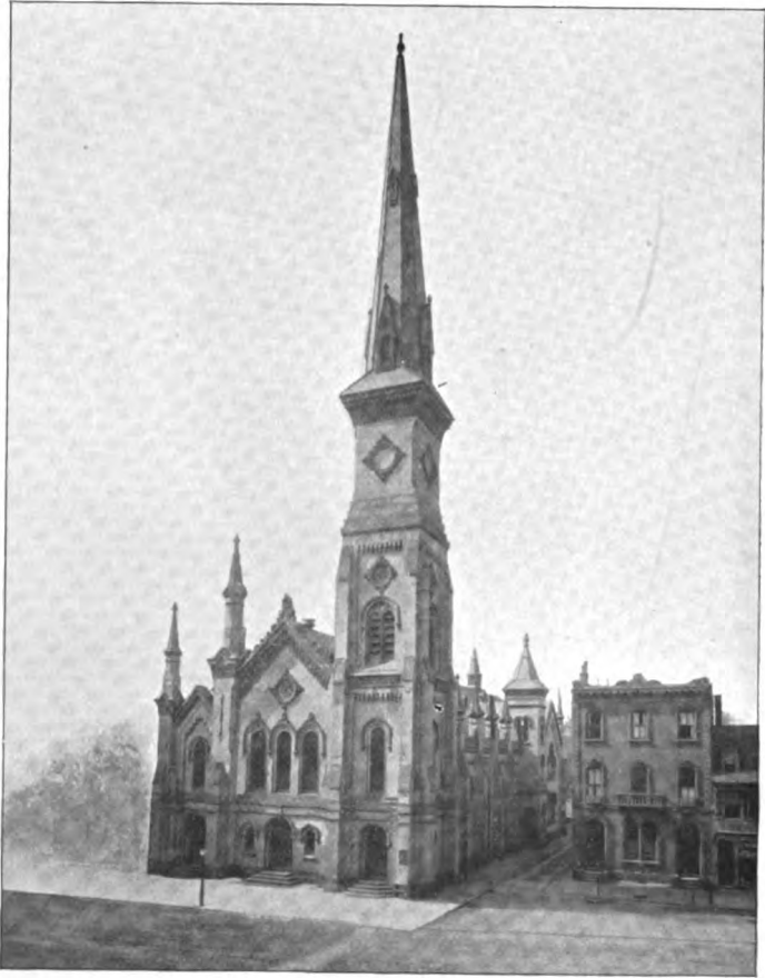
ENGLISH PRESBYTERIAN CHURCH. MARKET SQUARE. ERECTED 1858-59.
