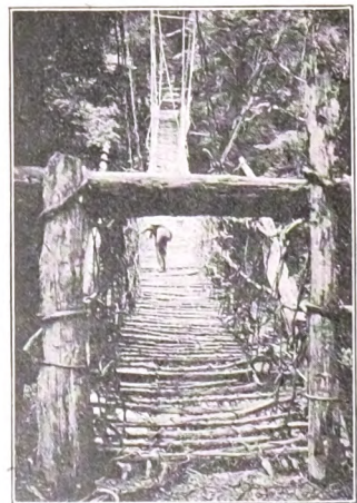
One of the many remarkable swinging bridges to be found in Japan. They are of almost unbelievable strength and durability.
