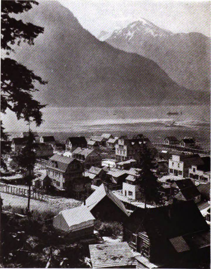
HYDER, ALASKA, ON THE PORTLAND CANAL
