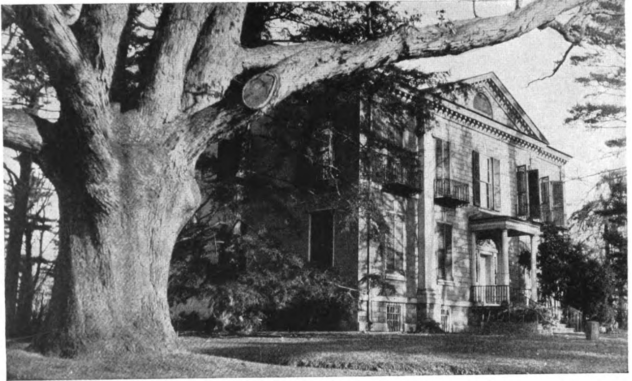
"THE HIGHLANDS," FORT WASHINGTON, NEAR PHILADELPHIA (Built in 1796 by Anthony Morris)
