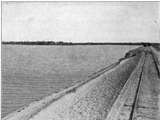
COLORADO RIVER LEVEE
