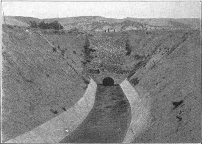
WEST PORTAL, GUNNISON TUNNEL, COLORADO
