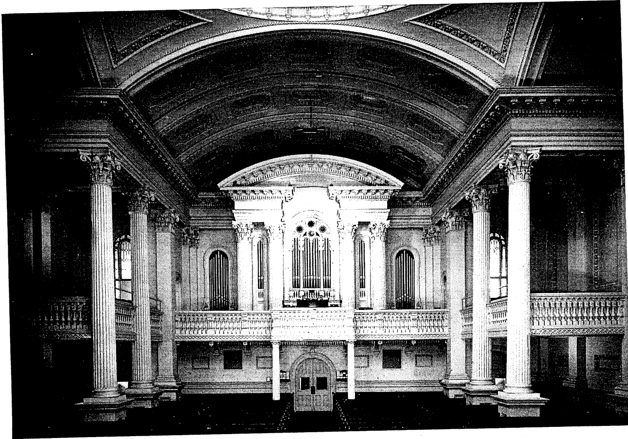
ARCH STREET PRESBYTERIAN CHURCH, PHILADELPHIA, PENNSYLVANIA
