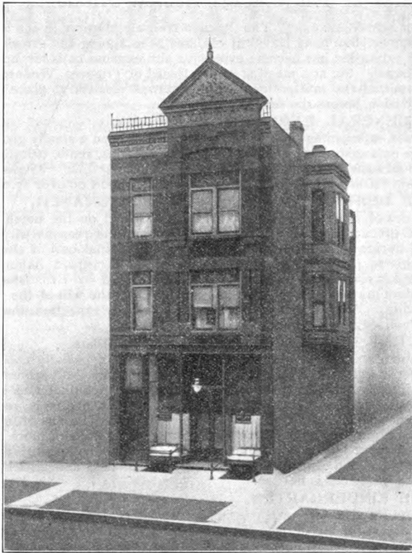
THE NEW WEST DIVISION STREET BRANCH. 326 West Division Street
