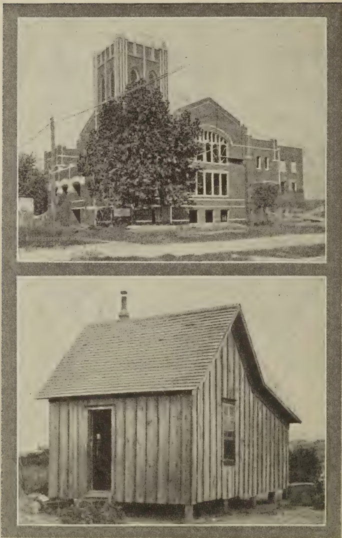
Above —The new church at Hugo in process of erection. Below —Manse at Hugo, Okla., occupied by Rev. R. P. Walker while he built four churches.
