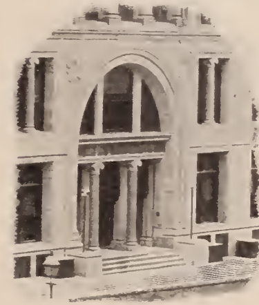
ENTRANCE TO THE HEADQUARTERS.
