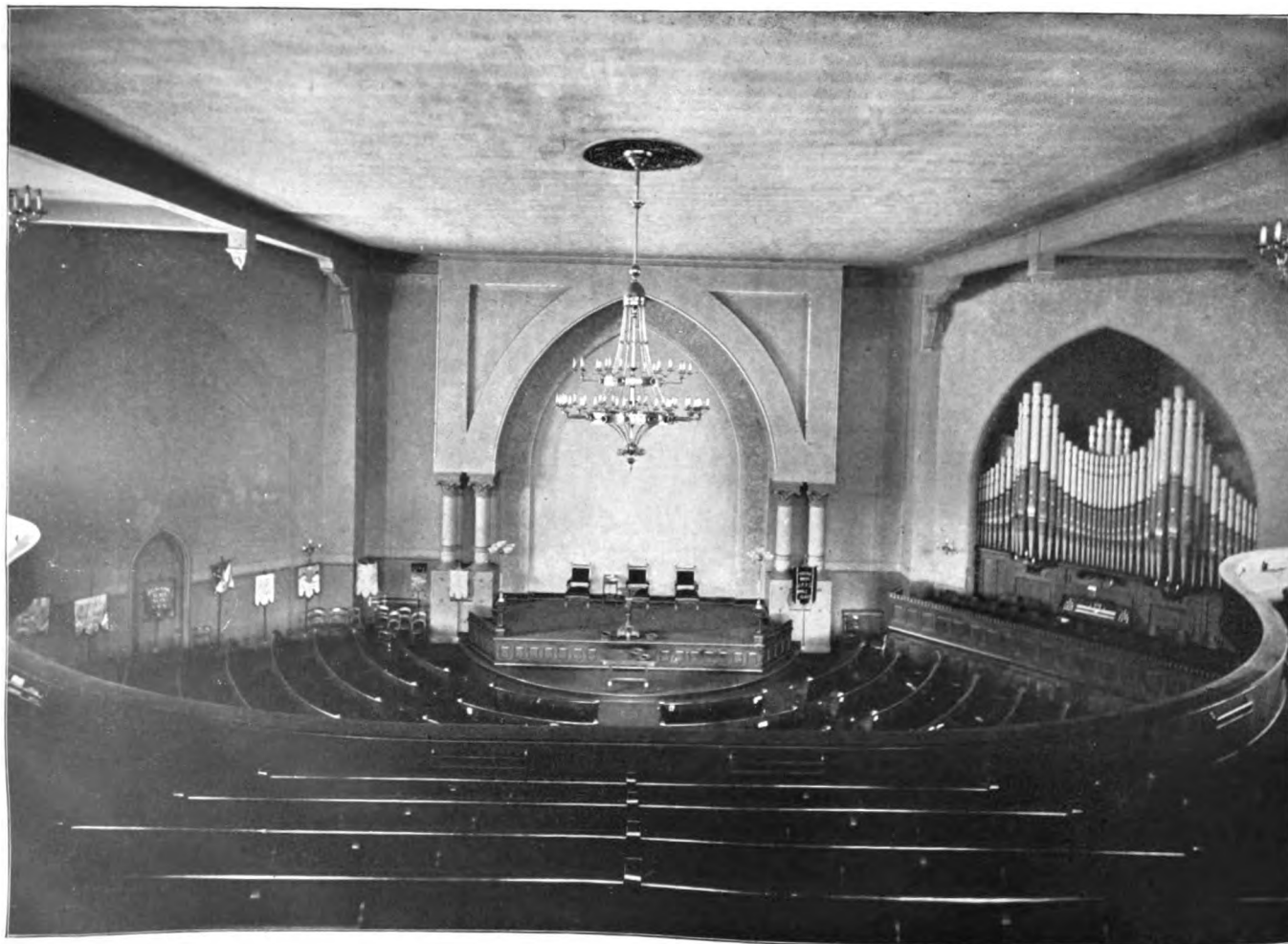
JEFFERSON PARK PRESBYTERIAN CHURCH—CHICAGO. (Interior View.)
