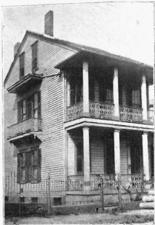
CHINESE MISSION BUILDING 223 South Roman St.
